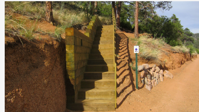
New trailhead steps and retaining wall, June
