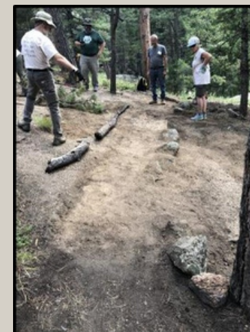
Built sustainable re-route for area's busiest trail
