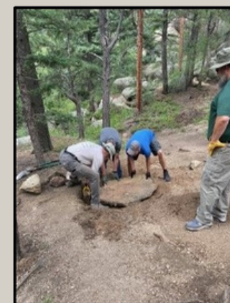
Designed re-route and emplaced rock
